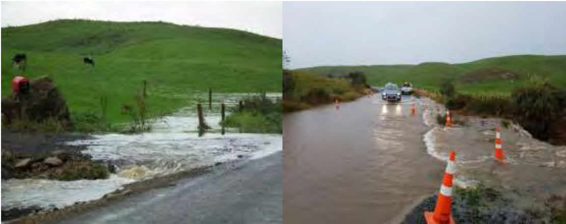
Run-off issues on conversions
