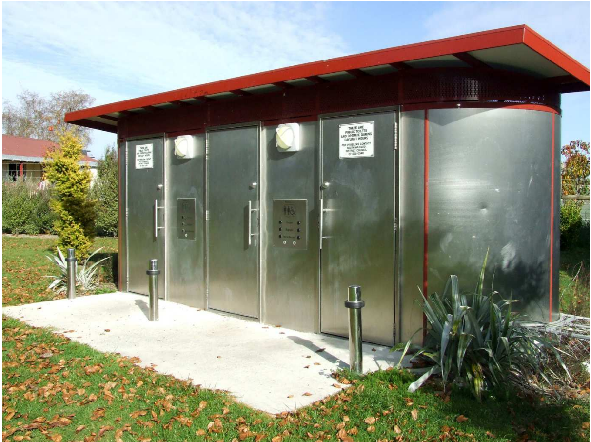
Tokoroa Youth Park toilets
