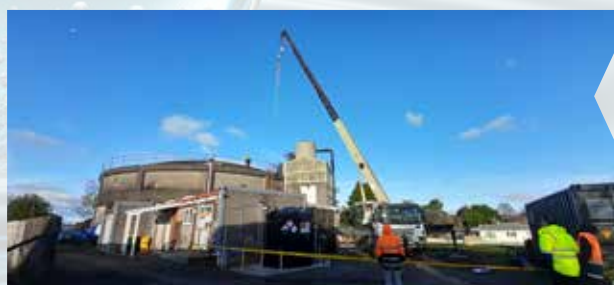
Service Engineers loading the new access ladder.
