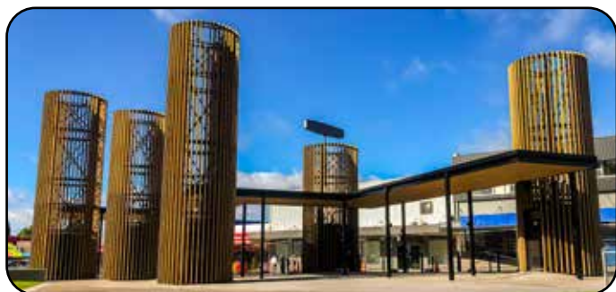
Above - the Leith Place toilet cylinders differ in heights and are joined by a covered walkway.
