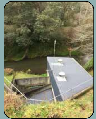
Spring and pump building located in Tīrau. The Oraka Stream is pictured in the background.
