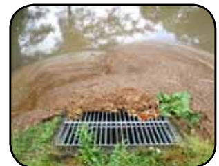
A close look at a detention dam in action.
