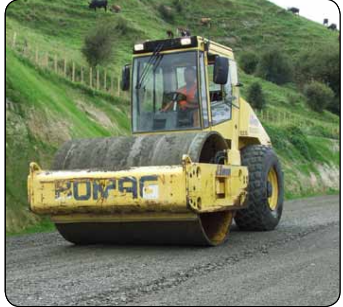
Part of the road rehabilitation process is when the roller compacts the road metal to form a hard surface.
