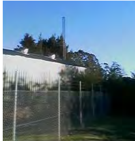
SWDC Hydrostatic Loop installed at some wastewater pump stations
