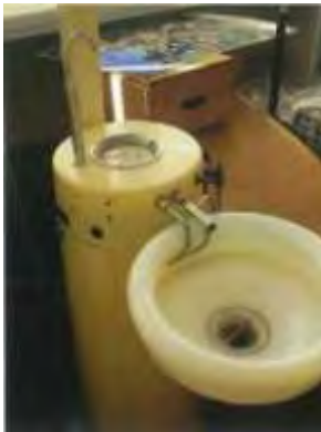
Dental cuspidors with inlets below the flood rim allow potential contamination
