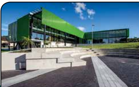
Toi-Ohomai Health and Science Building
