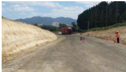
Traffic running through the new section of Old Taupo Road.
