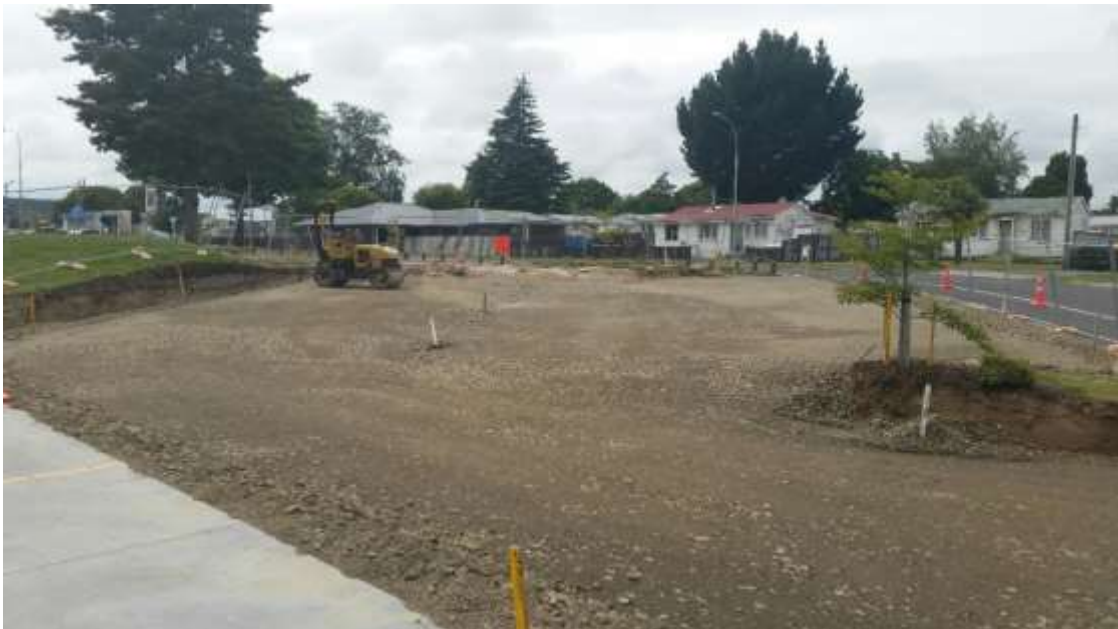
Development of the new carpark as of 23 December
