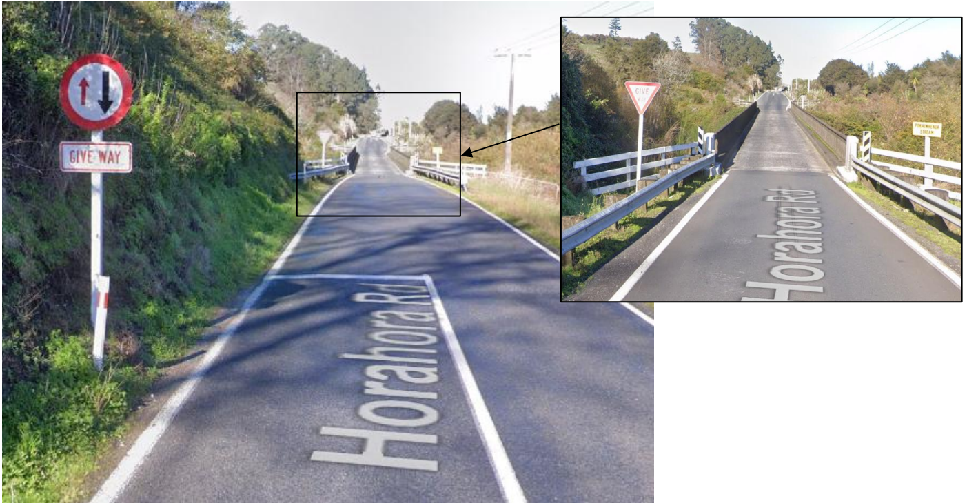
Figure 1 - Pokaiwhenua Stream Bridge, looking south
